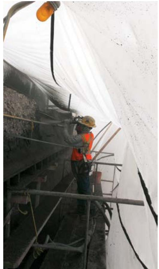
*Fig. 6: Shotcrete placement inside a heated bridge enclosure*
